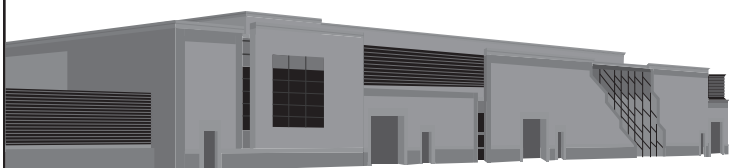
Tertiary Treatment building
